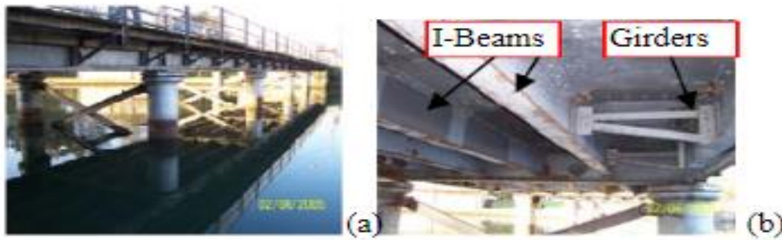
Figure 2-(a) An example bridge; (b) Part of the bridge structure
