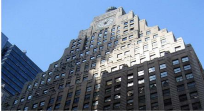
The paramount building at New York, United States [Source: https://untappedcities.com/ ]
