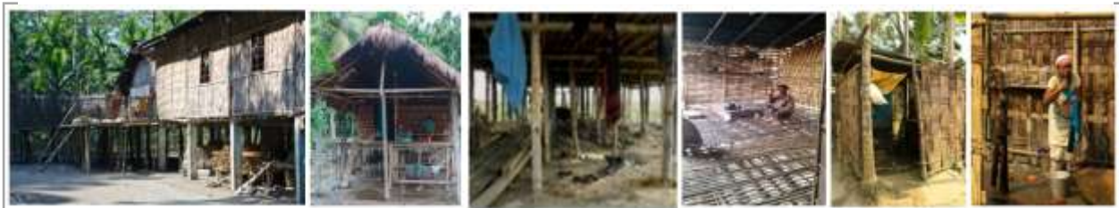
Figure 21 – Typical Deuri Tribe House – Pig stay &duckary under stilt, perforated floor and detached toilet.
