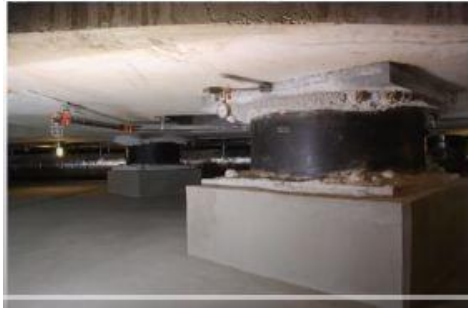
Figure 1:- Base Isolation System.
