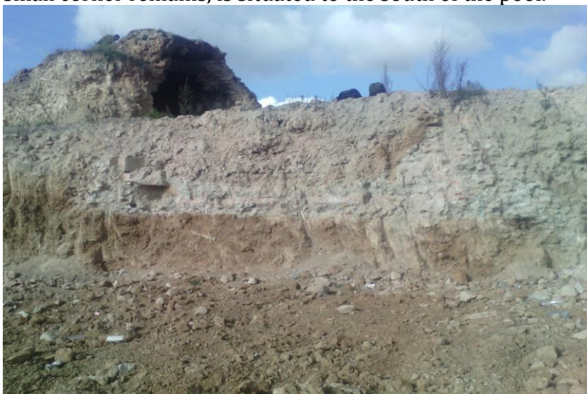
Fig. 11 The remaining part of the swimming pool
